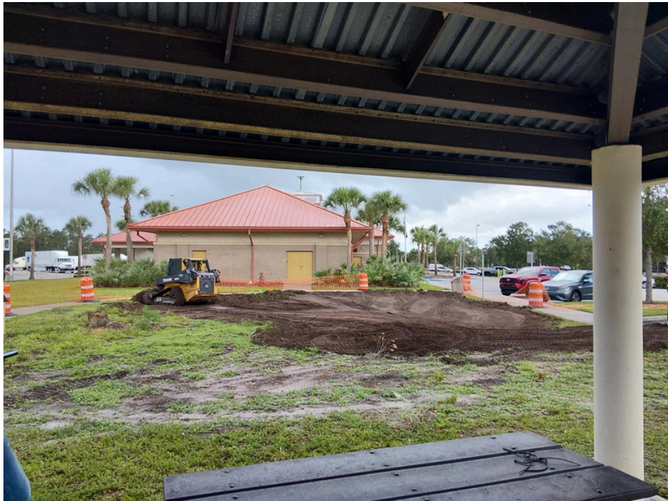
Interior soil graded and perimeter curbing formed, with caution tape and barrier barrels staging the work area.
